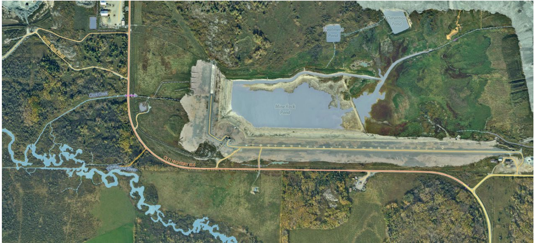
Figure 4- 4: Mine Rock Pond and Dam (Dec. 2023)
