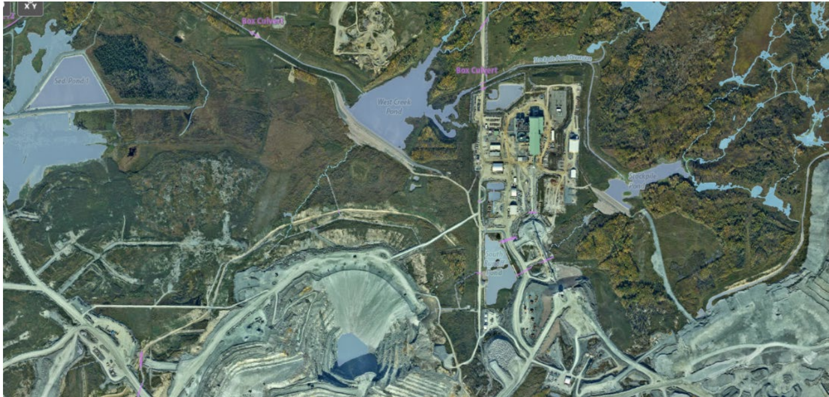
Figure 4- 3: West Creek Division and Plant Site Ponds (Dec. 2023)
