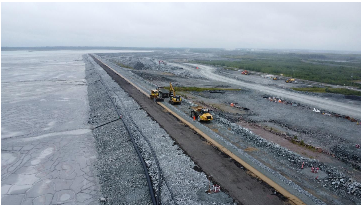
Figure 10. TMA Dam construction during filter placement, 2024
