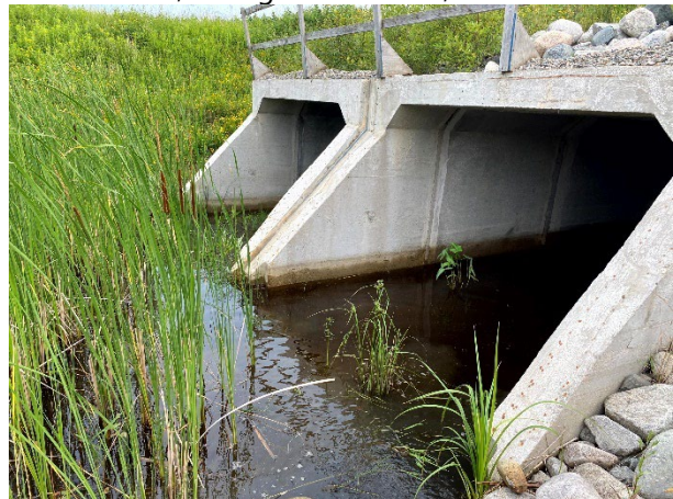
SPDC-01, Facing downstream, 2024-07-26
