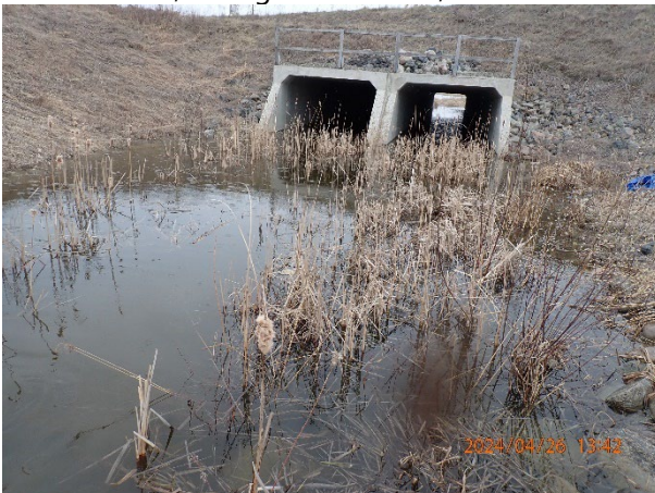
SPDC-02, Facing downstream, 2024-04-26
