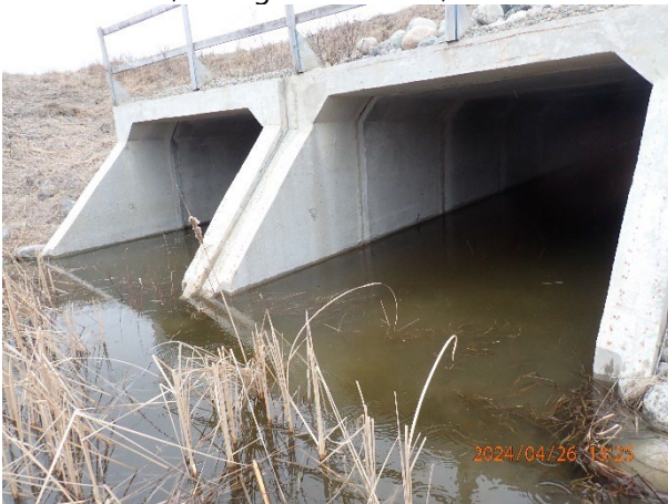
SPDC-01, Facing downstream, 2024-04-26
