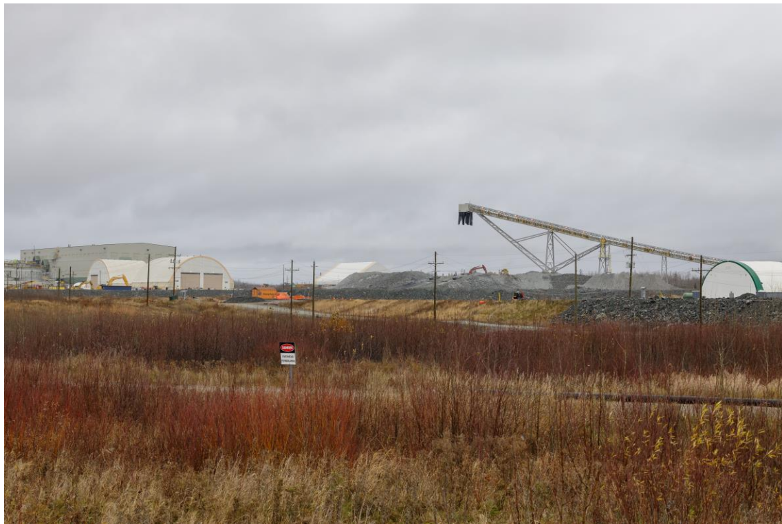
November 2024. Plant site area, all buildings have been removed.
