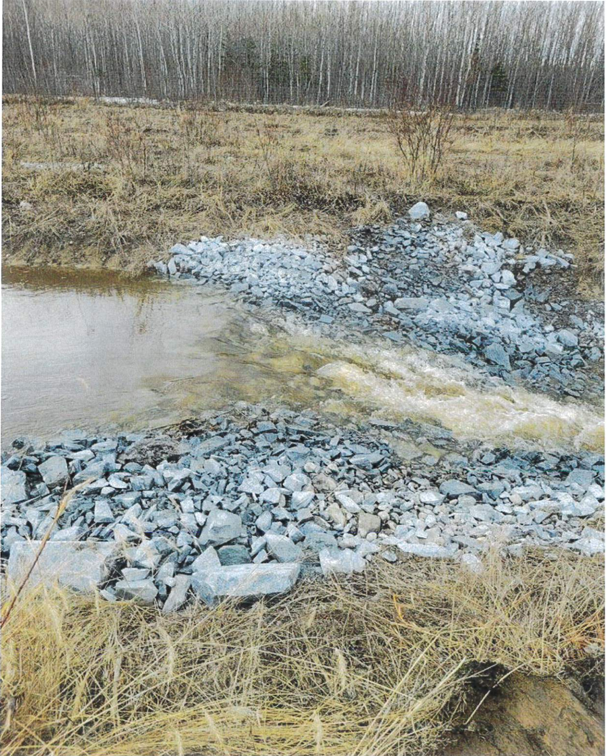
Photo 5: New rock check dam
