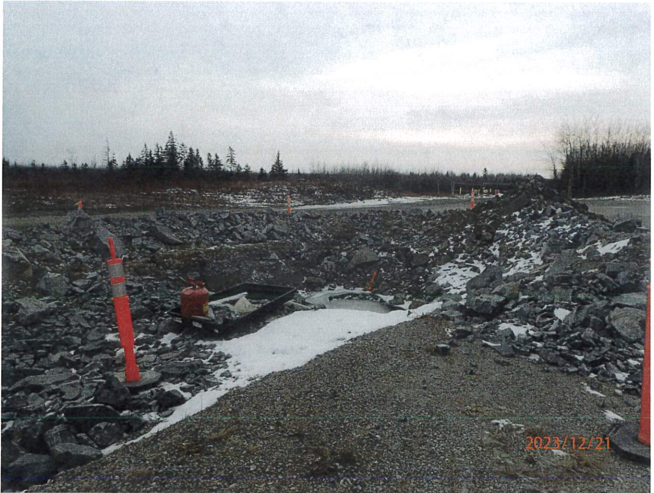
Figure 2: Collection sump constructed at seep location.
