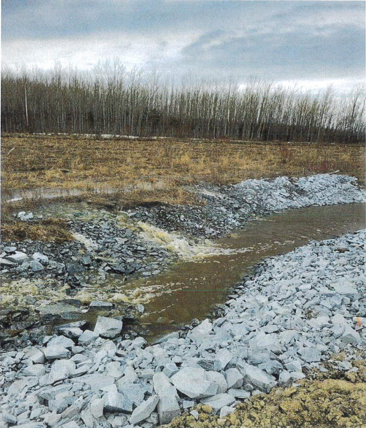
Photo 4: Marr tie-in repair
