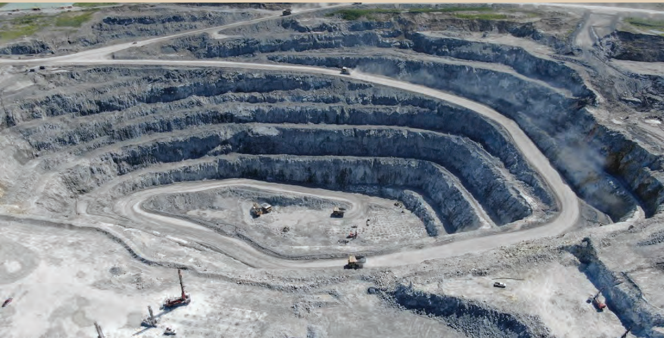
Aerial view of open pit; from surface to the pit floor is approximately 173m
