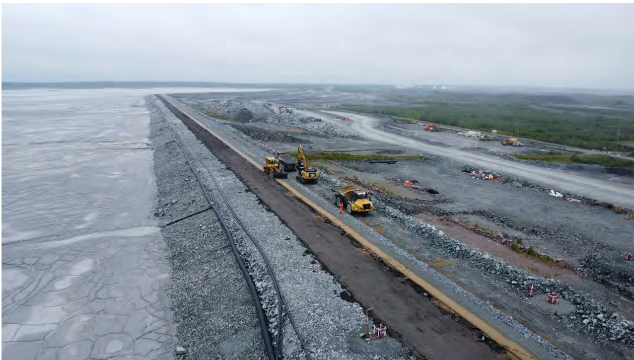
Figure 10. TMA Dam construction during filter placement, 2024
