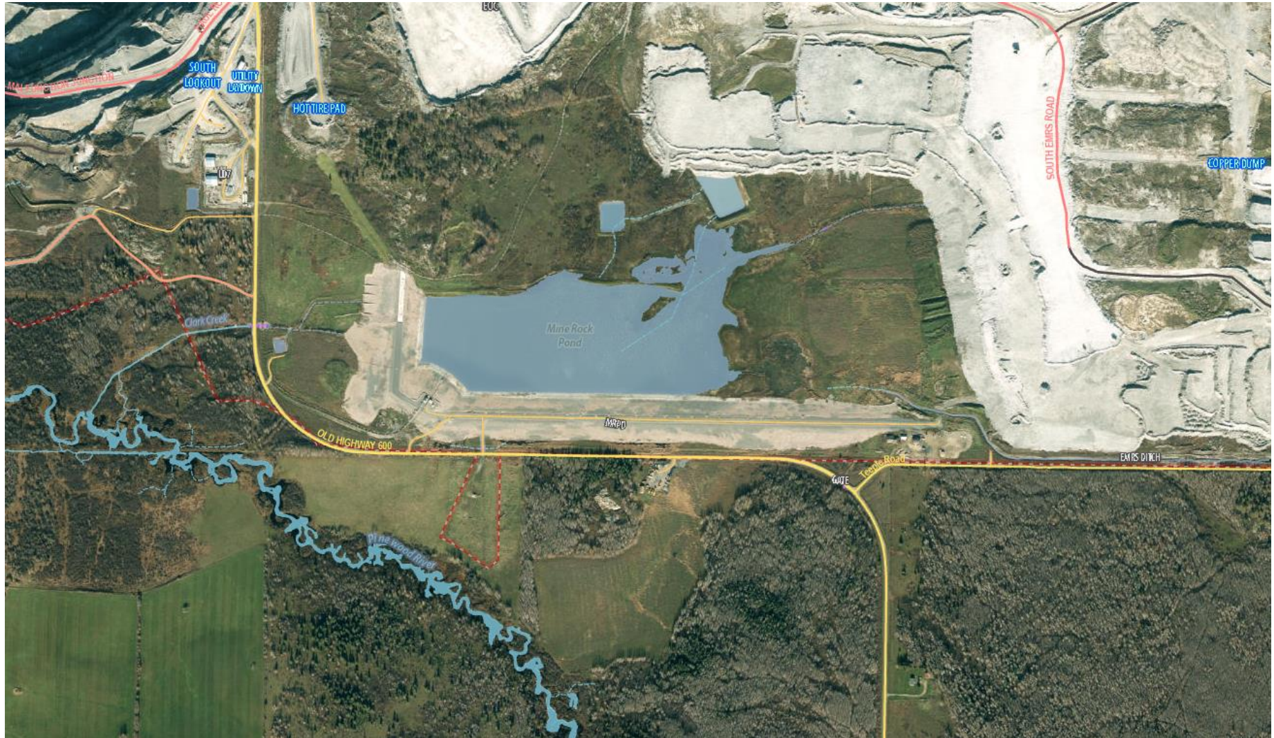
Figure 4- 4: Mine Rock Pond and Dam (August 2021)
