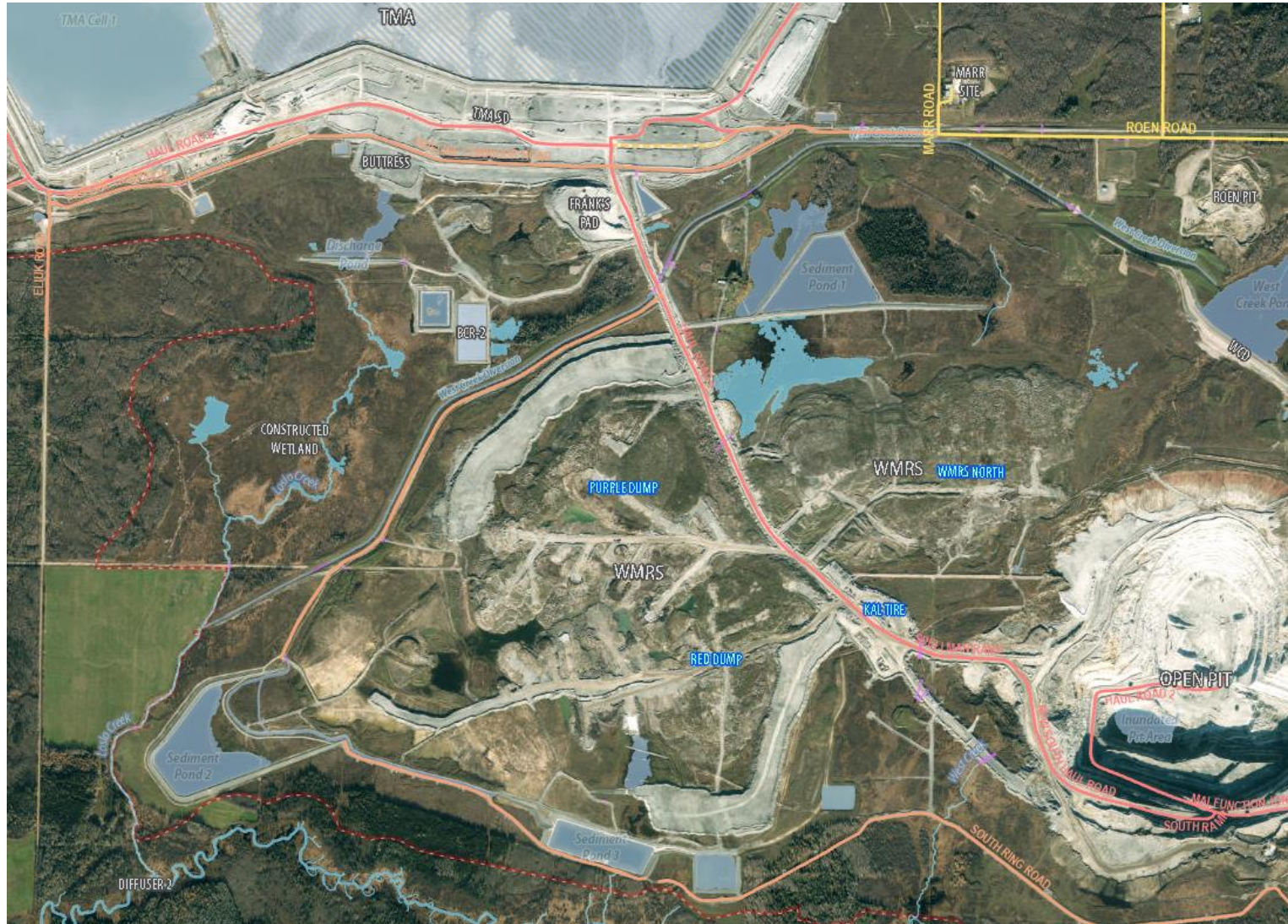
Figure 4- 5: Sediment Controls (August 2021)
