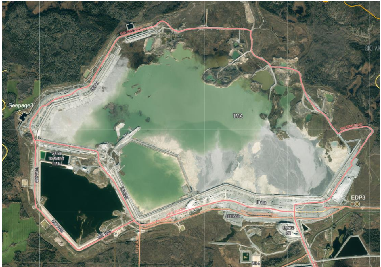
Figure 2 Seepage3 and EDP3 locations around Tailings Management Area.
