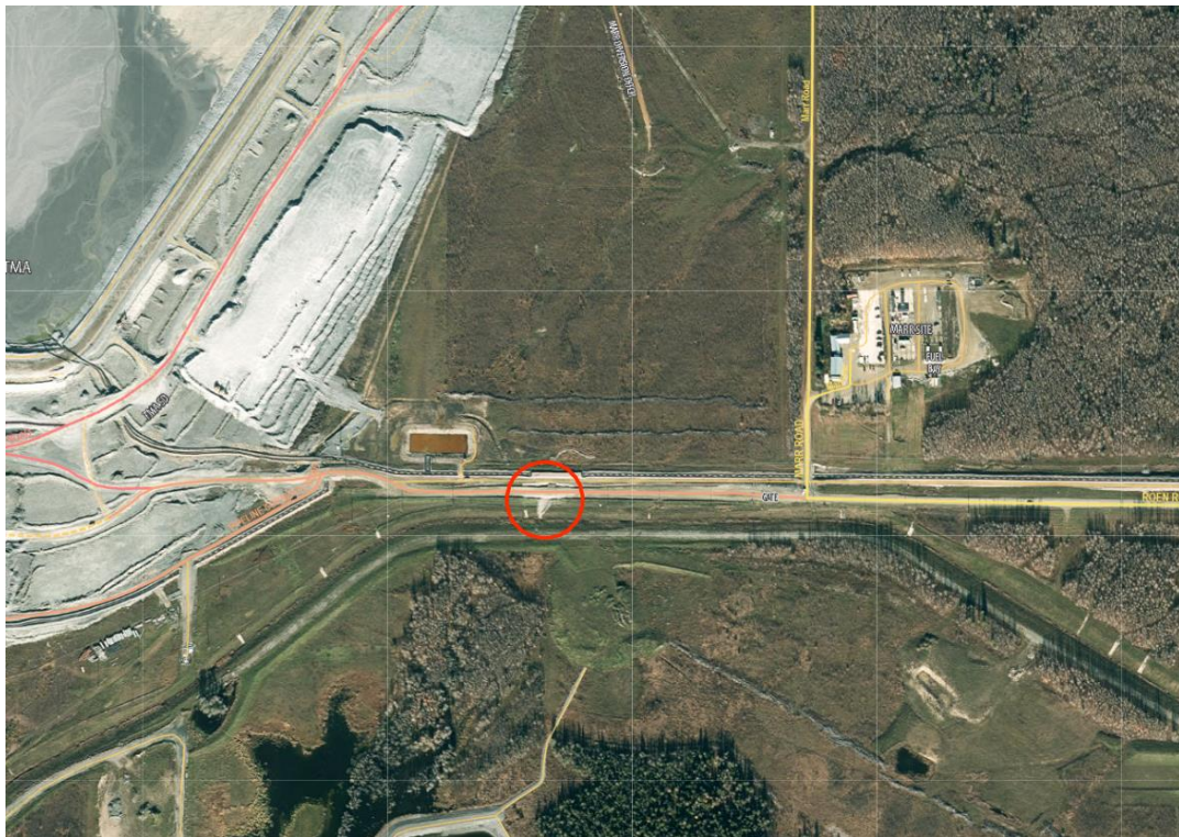
Figure 1 Location of turbid water observed travelling through culverts under Roen Road into West Creek Diversion.
