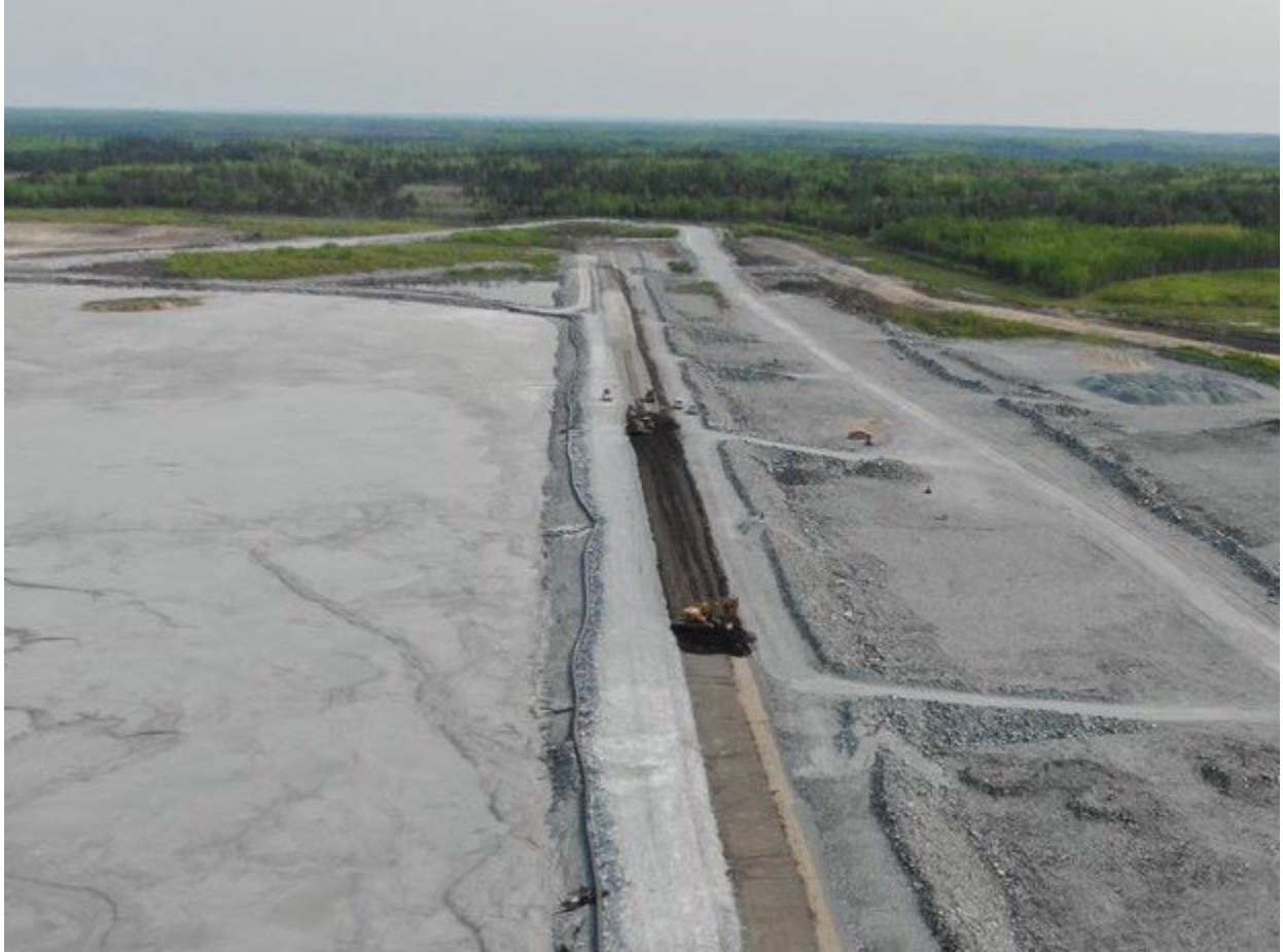
Figure 12. TMA West Dam 6 Construction 2023
