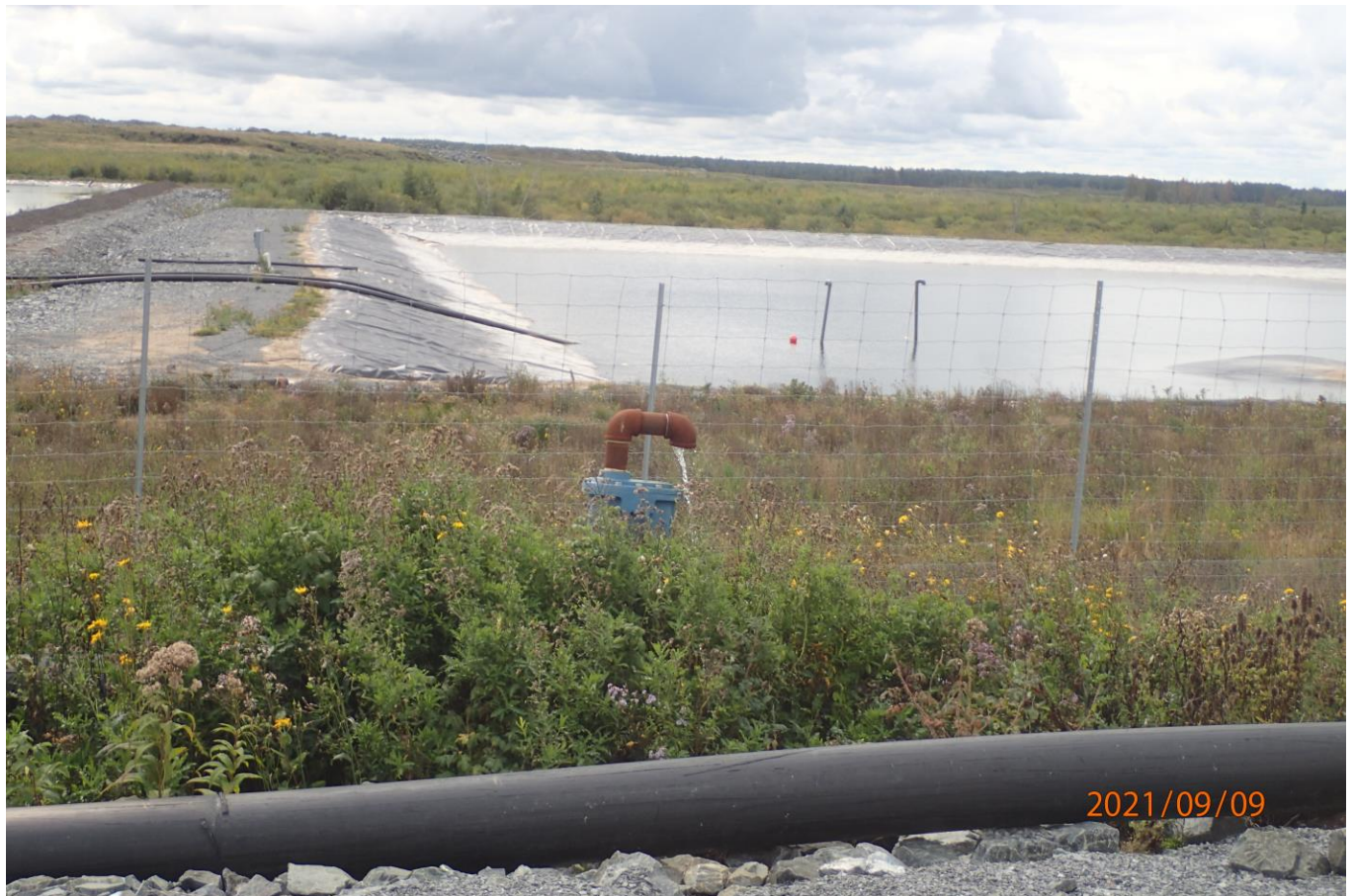
Photo 1: Leaking valve.
