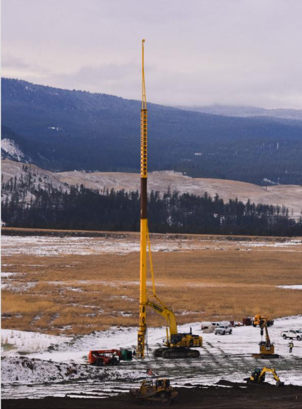
As we get closer to initiating mining of the B3 resource, stabilization work of tailings storage facilities has been a primary focus. At the New Afton Tailings Storage Facility (NATSF), where our mill tailings are stored, dewatering well trial work is ongoing. Dewatering is the primary method of facility stabilization – the less flowable the tailings material, the more stable the facility.
