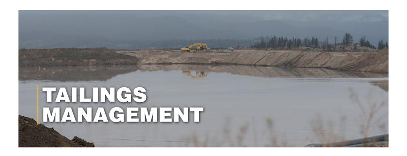
Tailings are a common by-product remaining following the extraction and recovery of valuable minerals from mine operations. They are generated by the milling process and are a mixture of finely ground sand- to clay-sized rock particles, water and processing reagents.
