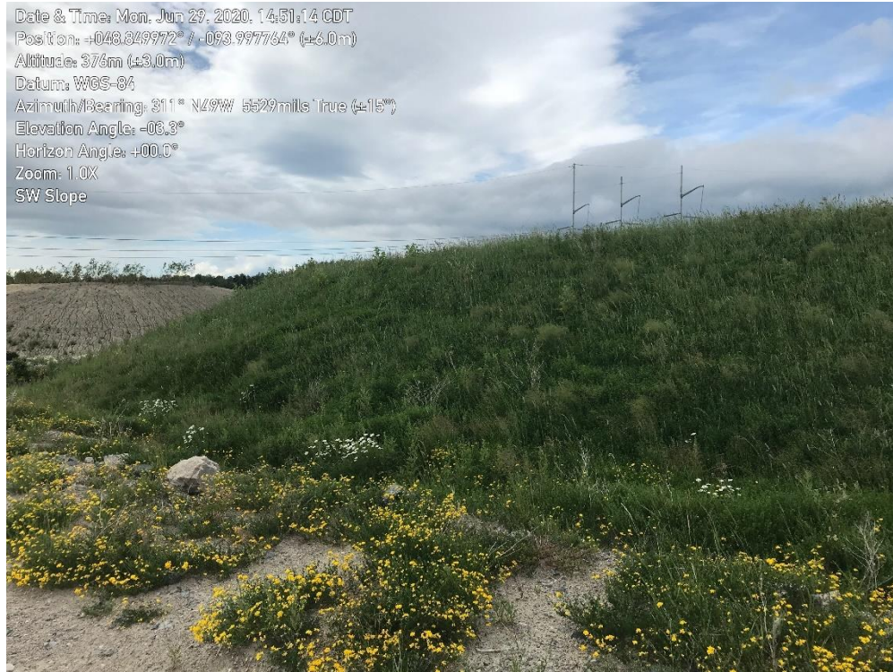
Photo A.5: Trial #1 slope overview showing established vegetation, looking West. June 30, 2020.
