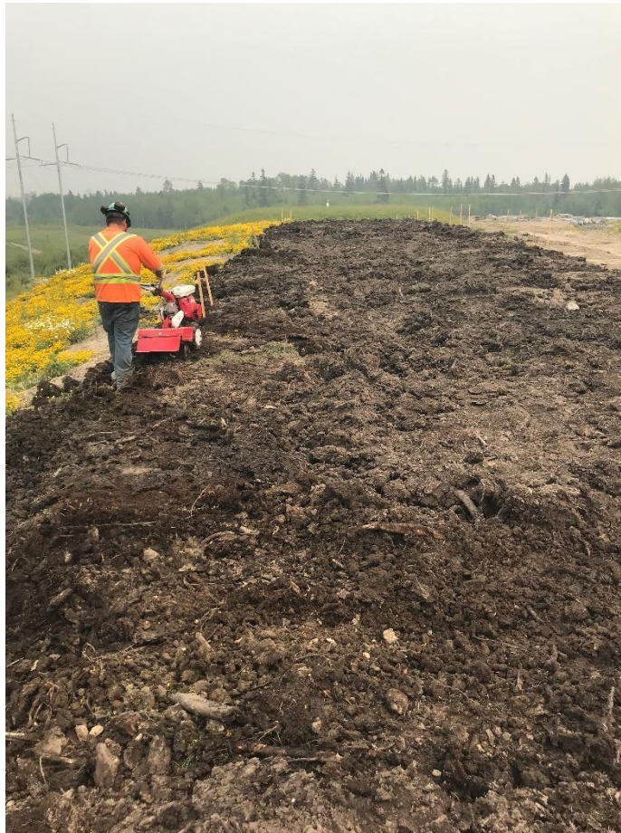
Figure 2: Initial effort at topsoil incorporation using a garden rototiller.
