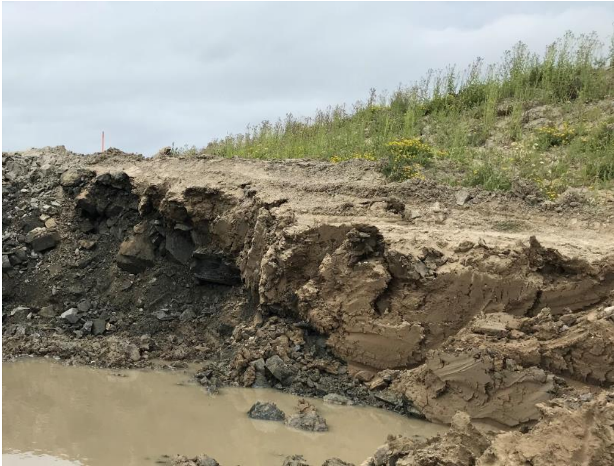
Photograph A.11: Borrow investigation of clay key layer on southeast corner of Trial #2. July 15, 2019.
