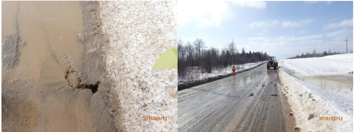
Figure 2. Eroded hole in Roen Road allowing turbid water from road to enter West Creek (left). Condition of road when mitigation measures were being installed by loader (right).
