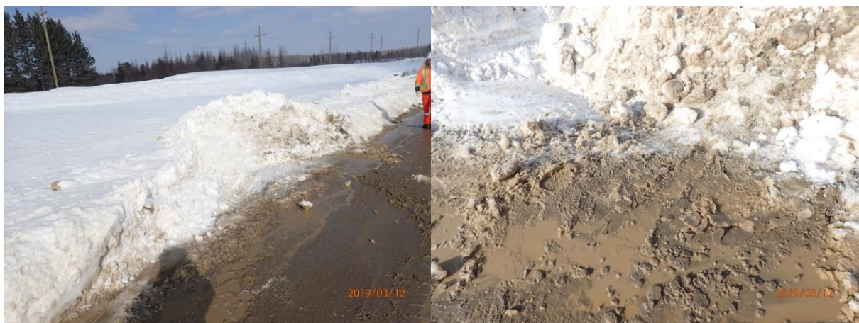
Figure 3. Punch out created on north side of Roen Road (left). Small swale made with shovel to help promote water-shedding from Roen Road (right).
