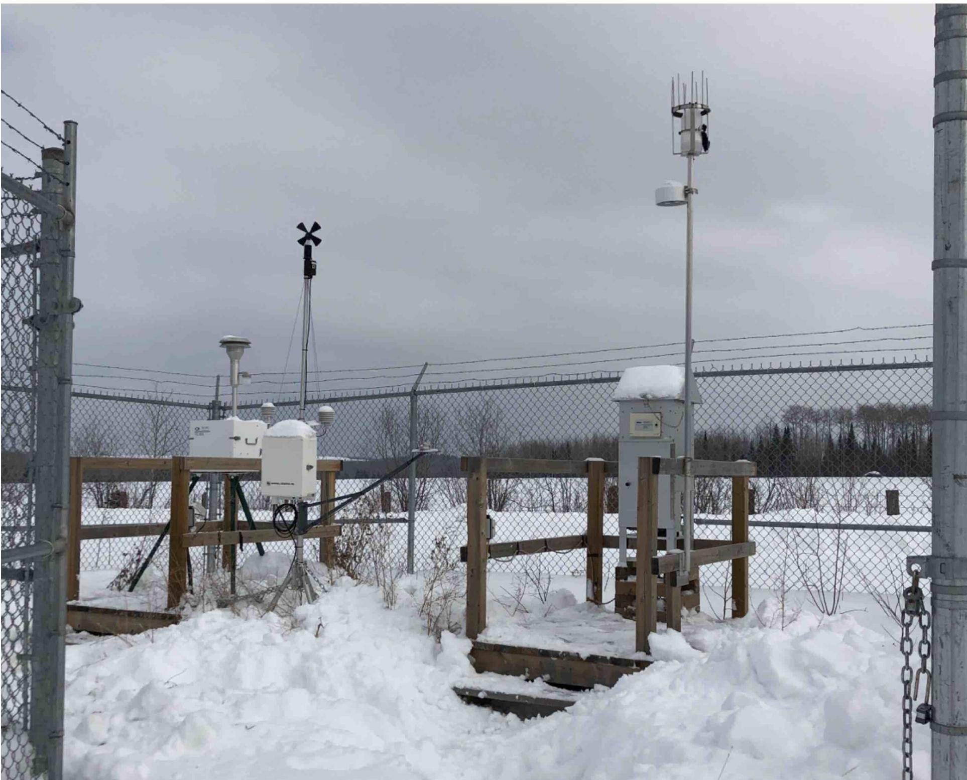
**Figure 2-4: Ambient Air Monitoring – Tait Road Station Air Quality And Meteorological Equipment**
