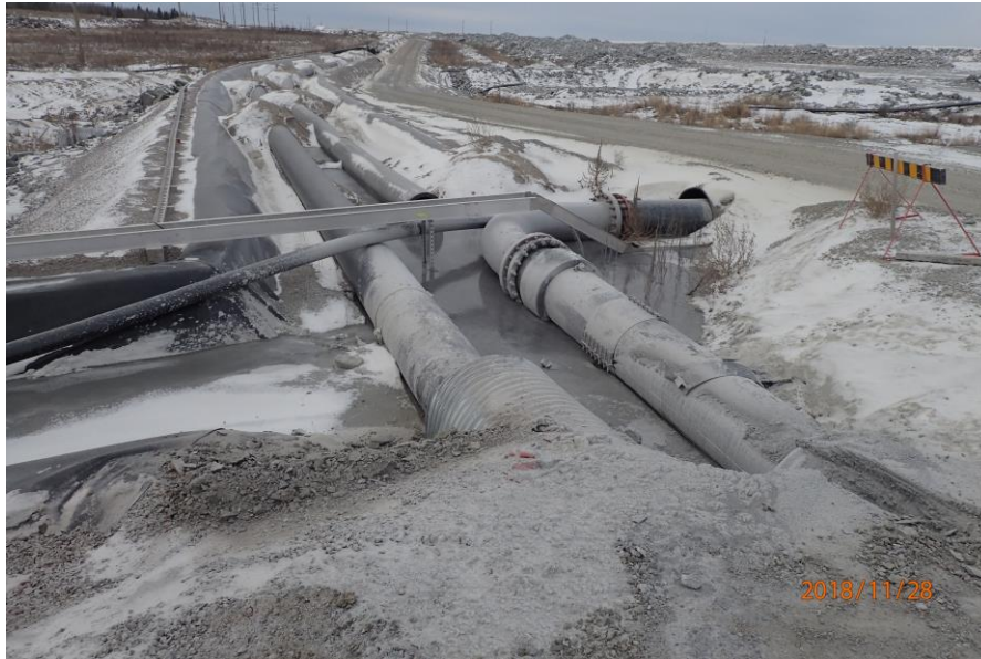
Figure 2 shows where the tailings sprayed out of the sleeve patch (lighter grey area along pipe) and ice build-up within the tailings corridor containment as a result of the spill.
