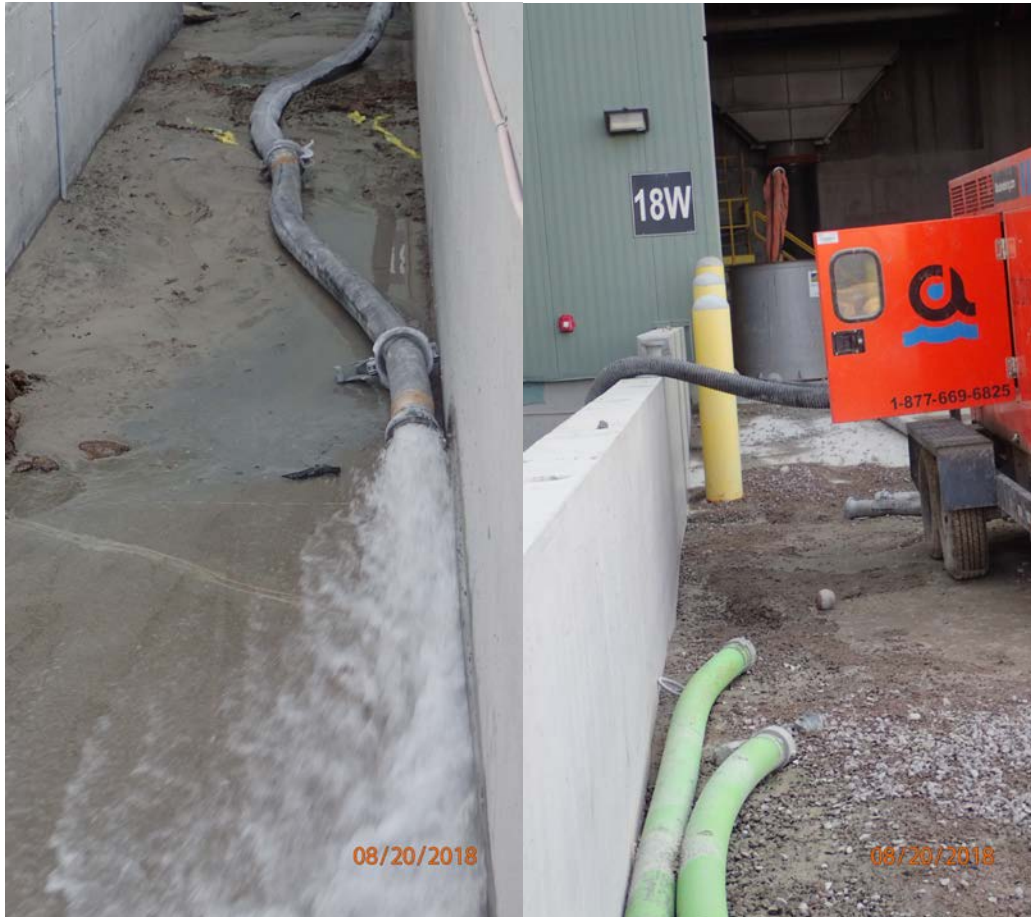
Photo 3. Black replacement hose on floor of containment area. Green hose line along containment wall.
