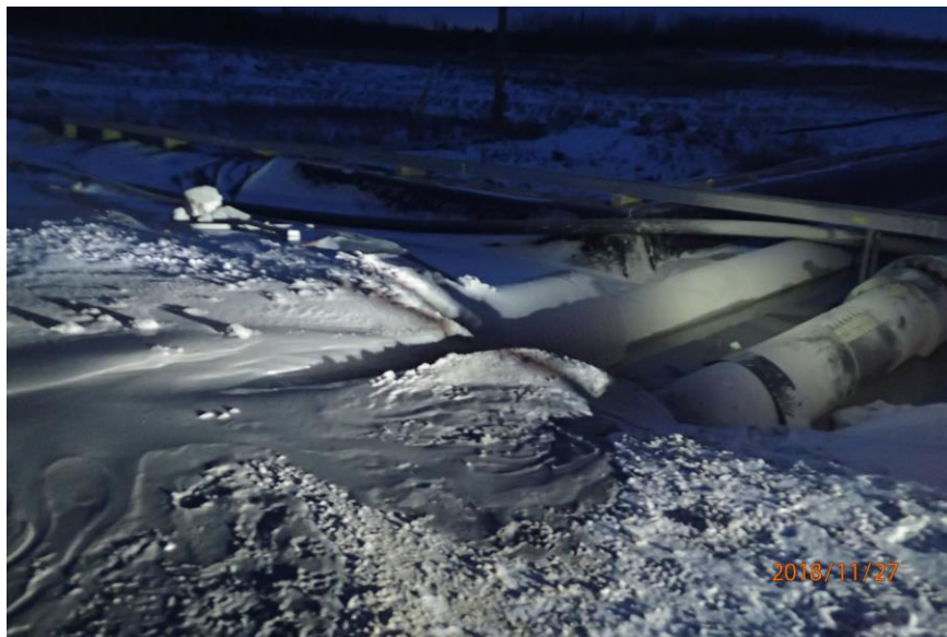
Figure 1 shows tailings leak location at 16:50. Tailings spilled onto access road to Emergency Dump Pond 6. Tailings also pooling inside containment due to ice build under WMP reclaim line.
