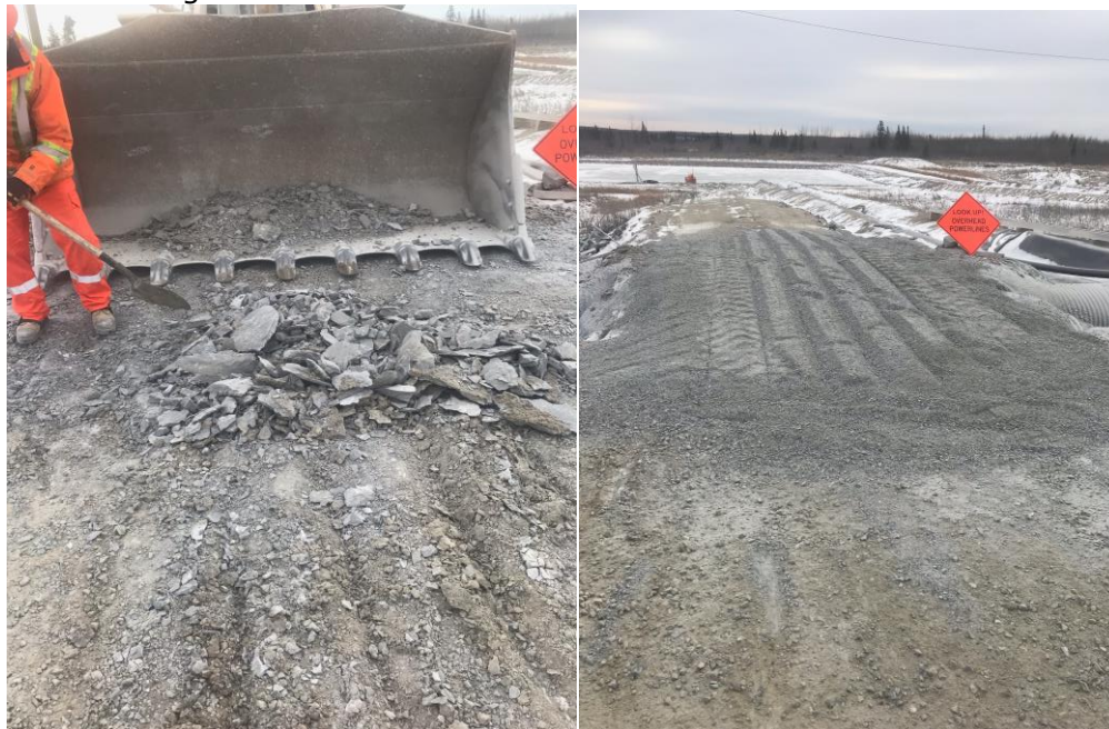
Figure 3 Shows removal of tailings and contaminated material as well as recapped road once clean-up was complete.
