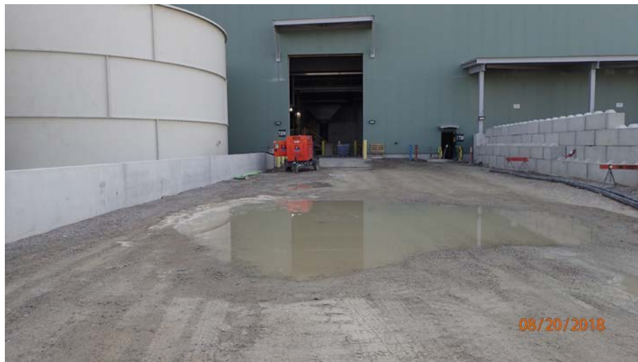
Photo 1. Extent of process water spill into truck alleyway of Door 18W.
