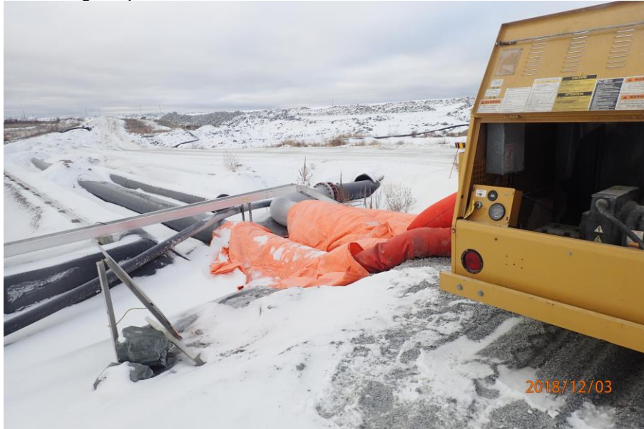
Figure 4 shows Allmond heater and insulated tarp being used to thaw the frozen tailings from the bottom of the containment as well as thaw ice dam underneath WMP Reclaim line.
