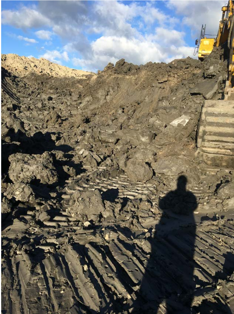
Photo 2 – Spill location after removal of affected clay
