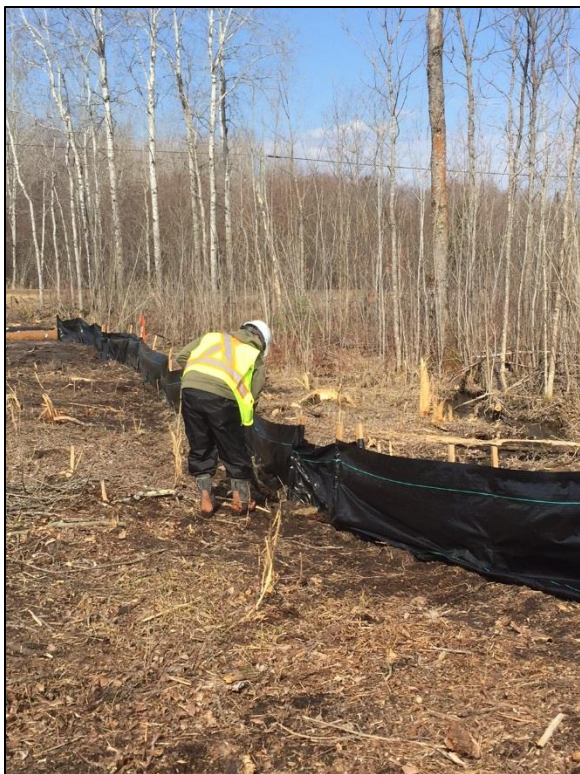
Silt fence installation (April 16, 2015):
