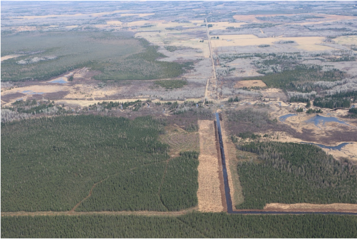
Highway 600 Re-alignment looking north towards the pinewood river showing root mat removal and side cast for the highway alignment and mulching of wood for the pipeline alignment to the west
