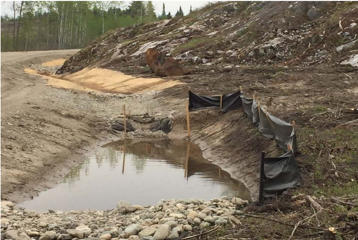
Standard sediment and erosion control measures including erosion blanket, check dams, sumps and silt fence
